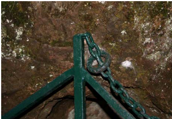
Diamond Cave: an integral chain passes through an eye bolt fixed in the rock above the gate – when locked, this stops the gate from swivelling on its single hinge
