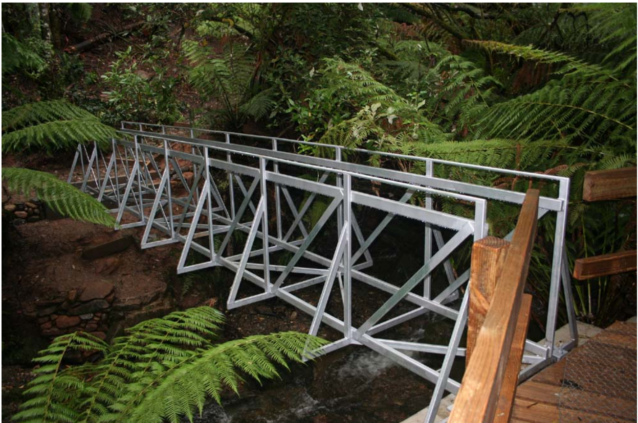
New bridge under construction on the Fern Glade track, Marakoopa Cave, Mole Creek
