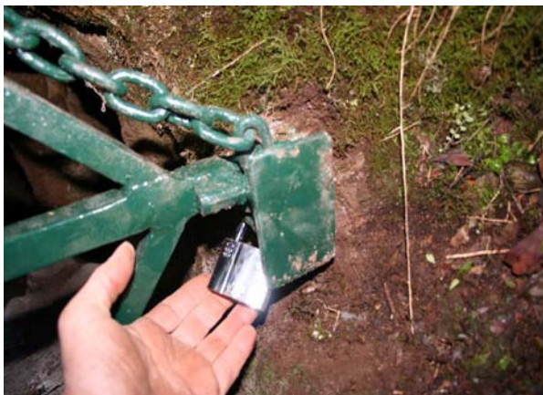
Diamond Cave: the chain passes through a second eyebolt at the locking point. The lock cannot be removed by cutting the chain.
