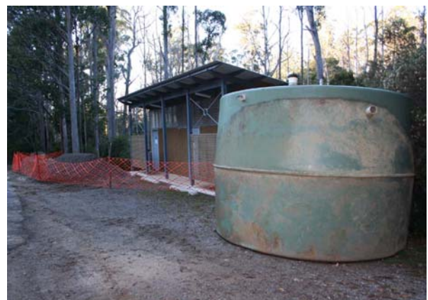
New amenity block at King Solomons Cave. The holding tank is shown waiting to be deployed following repairs to the site.
